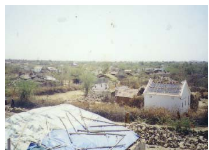
ESTCOURT HAILSTORM DAMAGE
